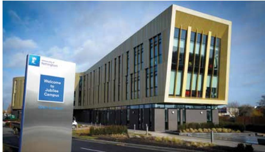
To create the high performance external envelope, EOS completed the design, engineering, manufacturing and supply of the infill walling Steel Framing System (SFS).
