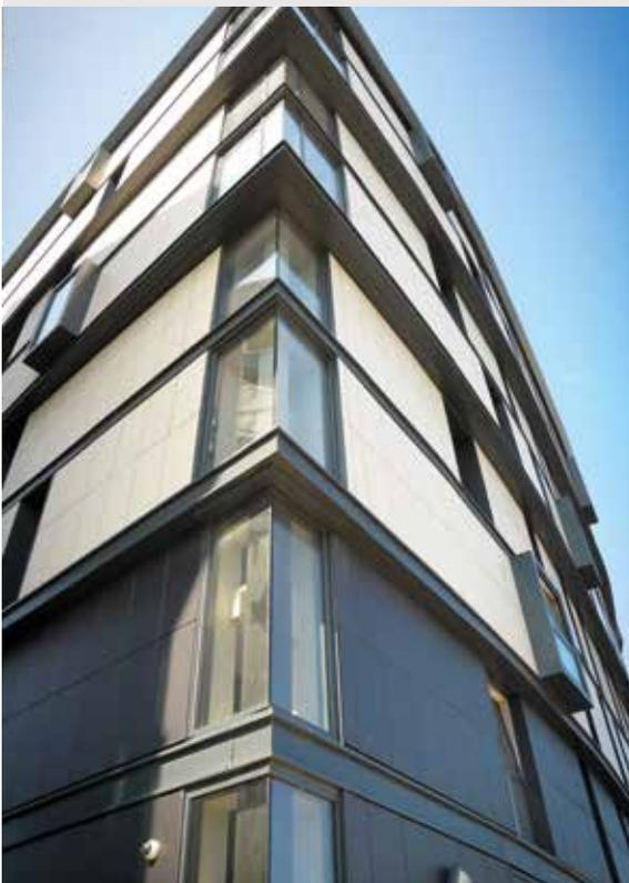
EOS designed and manufactured a light gauge steel infill framing system for the project together with overhang support plates for the extensive sweeping radius curve to front elevation. EOS engineered bespoke 'inside out fixings' for the internal head track and also used shot fired fixings.
