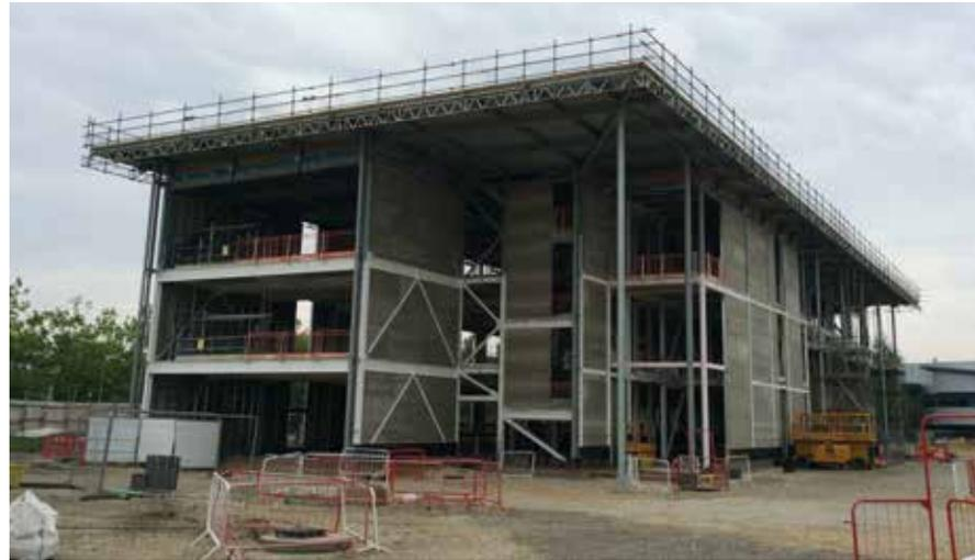
This early involvement enabled the installers to accurately price based on the complete design, offering Kier complete reassurance. EOS provided SFS infill to a hot rolled steel frame for the three floor building. This was also the first project where EOS utilised their slotted head track DHT product which not only halved the number of fixings required, but dramatically reduced installation time and risk on site.
