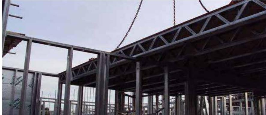
On the primary structure, EOS co-ordinated an engineered, load bearing framing system to interface with the poured and shuttered concrete main structure. This system is able to achieve high tolerance swings. EOS integrated both SFS infill to the concrete primary structure and infill to hot rolled feature box windows.
