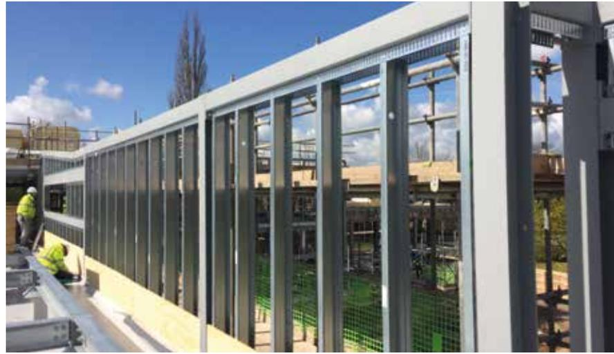
There were areas of brise soleil sun shading which were connected directly back to the SFS. EOS also specified additional pieces of steel to fit within the SFS sections in order to bolster the thickness and ability of the SFS studs and to support the load of the brise soleil.
