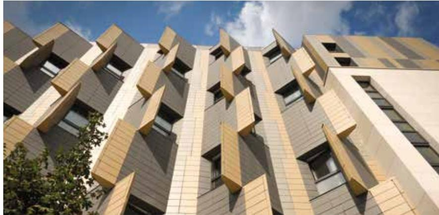
The tolerances and high-specification cladding system required all the technical insight of EOS to design and manufacture a fully offsite solution fixed to the main concrete frame, erected by main contractor Tolent.
